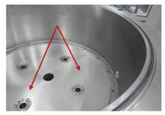
Fig.3: View of filter mesh installed on ANFD drier (coutrtsey M/s Hospira Pvt. Ltd. Chennai)
