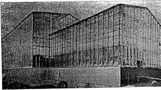
9 Dry working conditions achieved by temporary structure clad in plastic sheet
