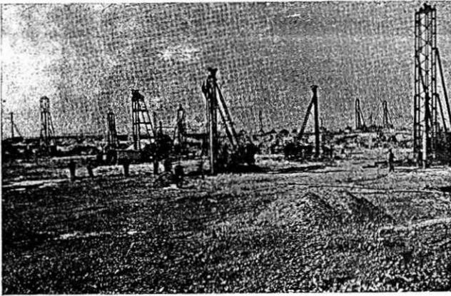
5 Corner of large steelworks site during piling operations, indicating amount of planning required to co-ordinate work of a large piling contract
