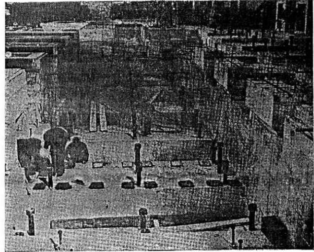
8 Mill foundations being prepared to receive the stands. Levelling pads being grouted in foreground
