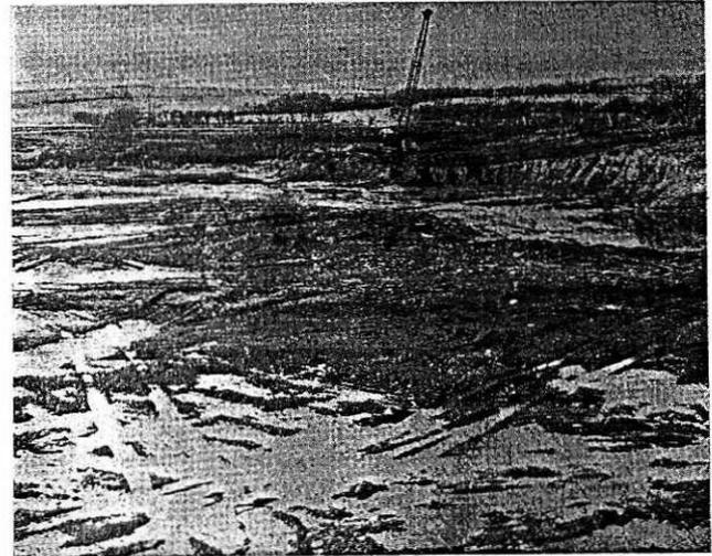
4 Early stages of site levelling. Up to 10m.yd<sup>3</sup> of spoil may have to be removed
