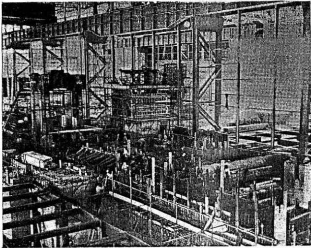
3 Typical example of complex rolling mill foundations
