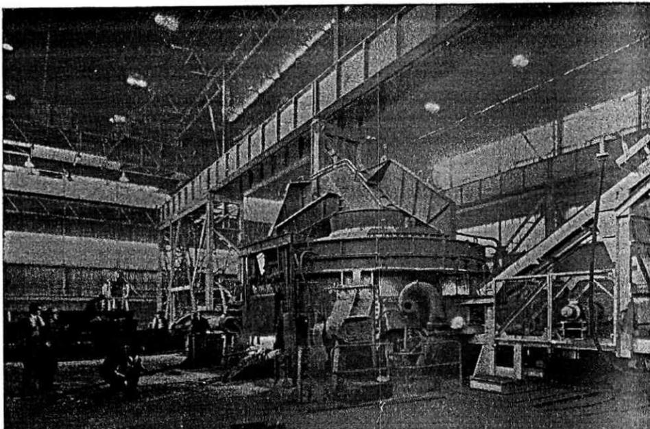
9 Fettling the prerefiner with lime powder
