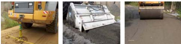
Figure 11. Construction of the experimental road section
