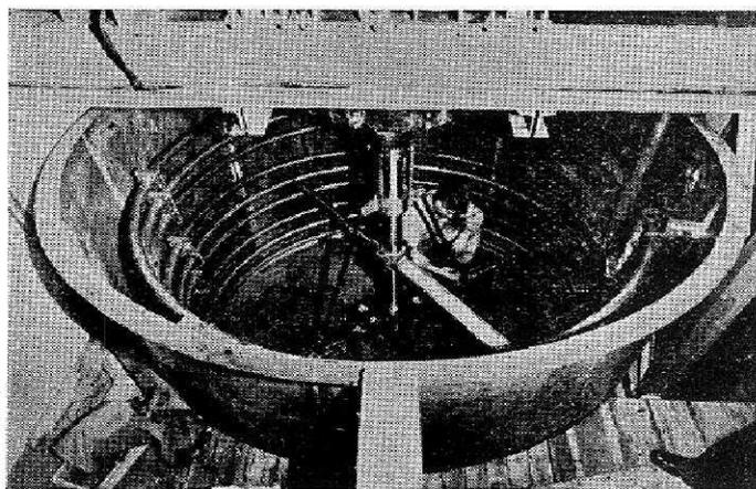
FIG. 4 — MONEL GRANULATING TANK FOR THE PRODUCTION OF POTASSIUM DICHROMATE (By courtesy of Chrome Chemicals Pty. Ltd., Parramatta, N.S.W.)
