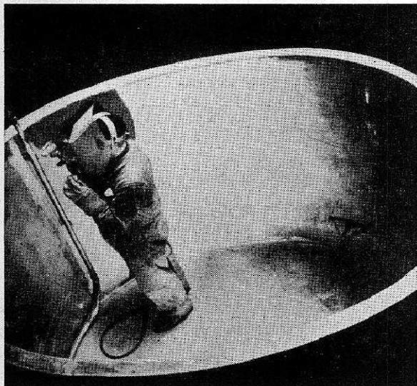
FIG. 11 — CARBON ARC WELDING OF MONEL TANK FOR USE IN INK MANUFACTURE (By courtesy of Welders Ltd., Belgium)
