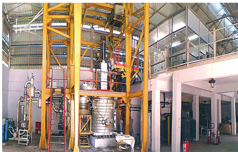
Fig. 1: Magnesium Pilot Plant facility at CSIR-NML
