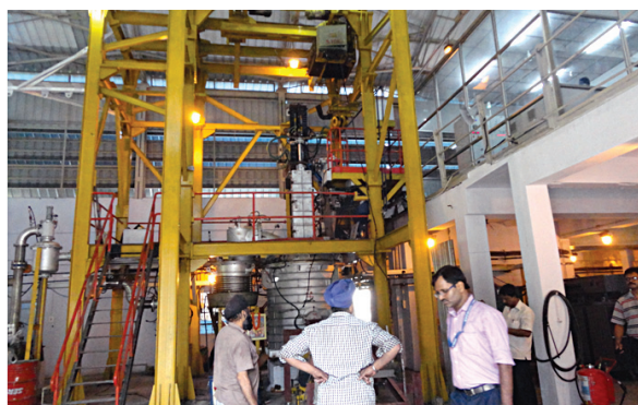
Developed Magnesium pilot plant
