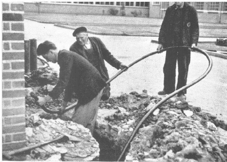
Fig. 5. Solidal cable being installed underground.
