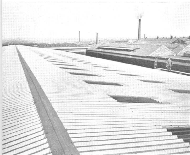
Fig. 2. Garage roof of Noral industrial aluminium sheet.
