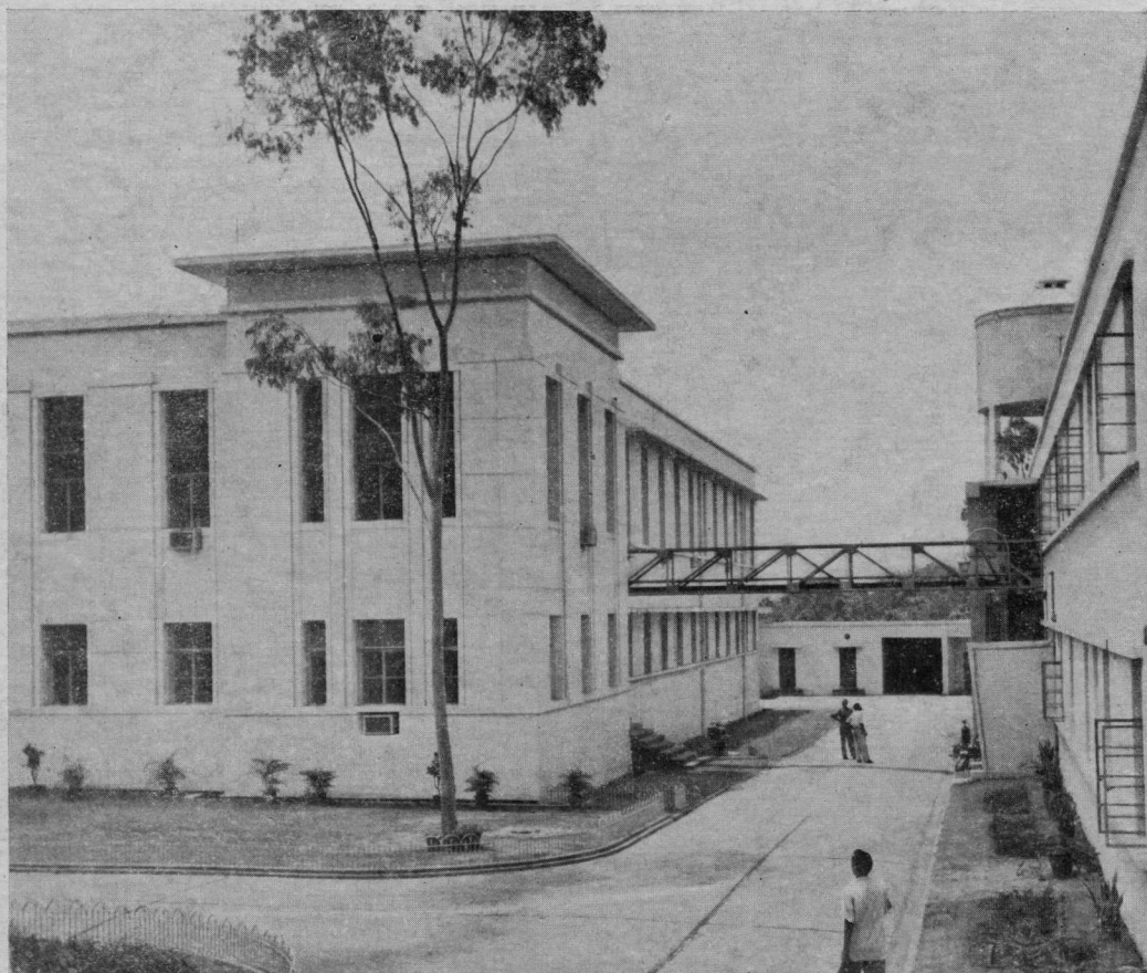
FIG. 71 — A VIEW OF THE EXTENDED WESTERN WING OF THE MAIN BUILDING OF THE NATIONAL METALLURGICAL LABORATORY
