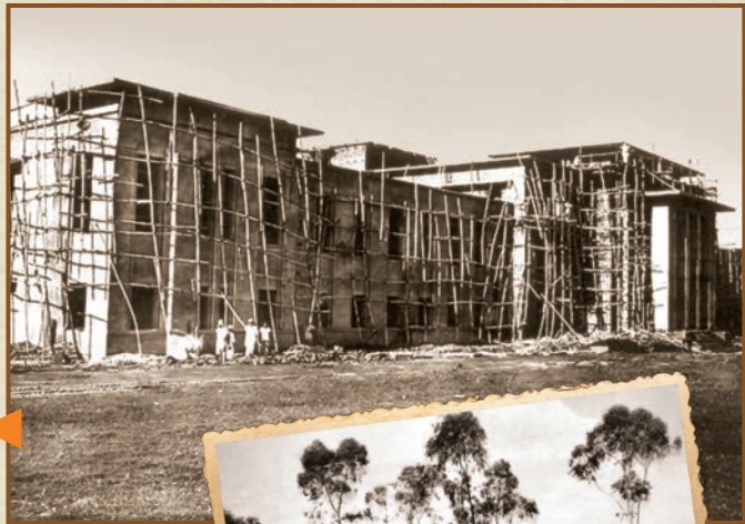
Construction work of NML building started
