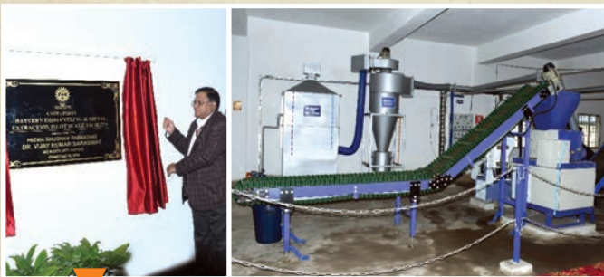
CSIR's First Battery Dismantling & Metal Extraction Pilot Scale Facility. Inaugurated by Dr. V. K. Saraswat, Niti Aayog
