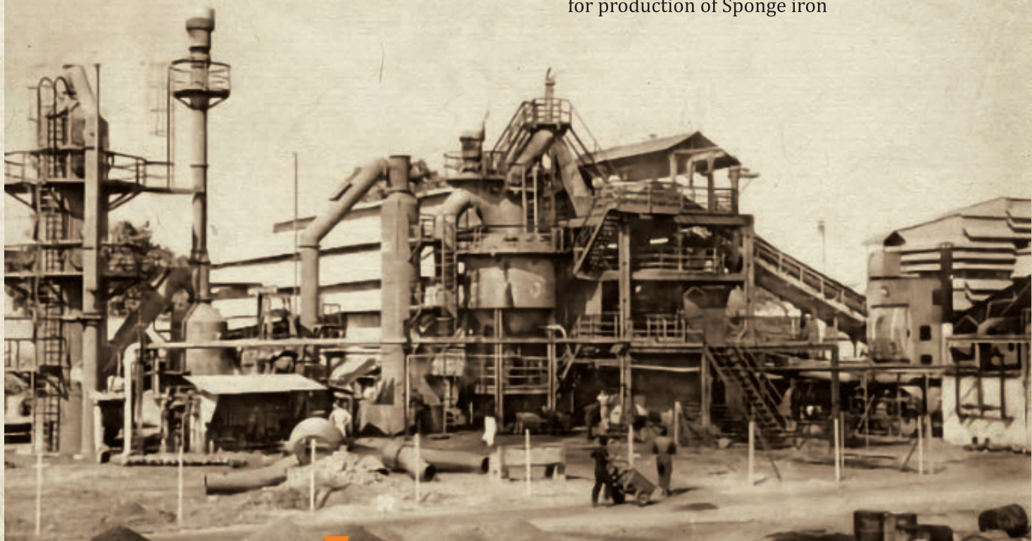
Sponge Iron Plant (Low Shaft)
