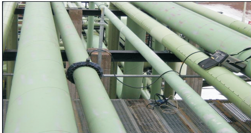
Fig. 4: Guided Wave Inspection On a pipeline.
