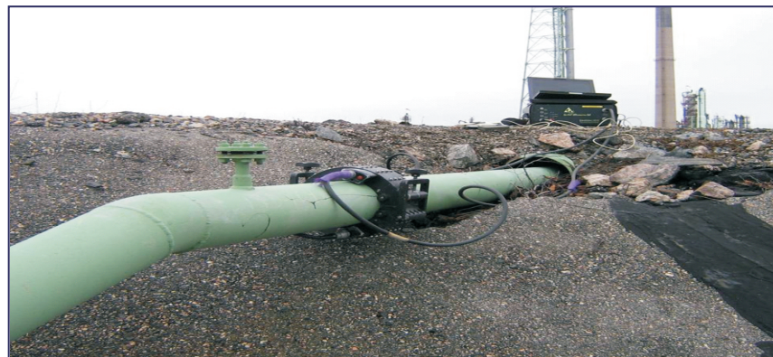
Fig.5: Guided Wave inspection on a road crossing piping.
