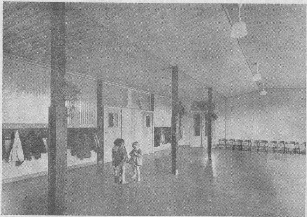
3 Aluminium false roof
