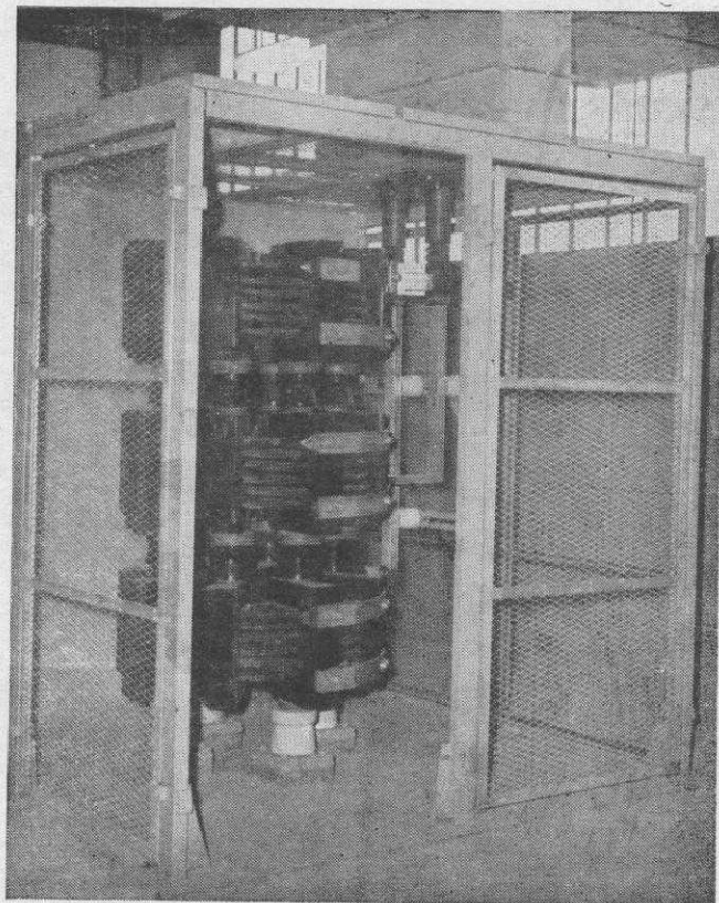
10 Dry-type reactor wound with aluminium stranded conductor, operating in a large French generating station
