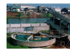
Clariflocculator (In Effluent Treatment Plant)
