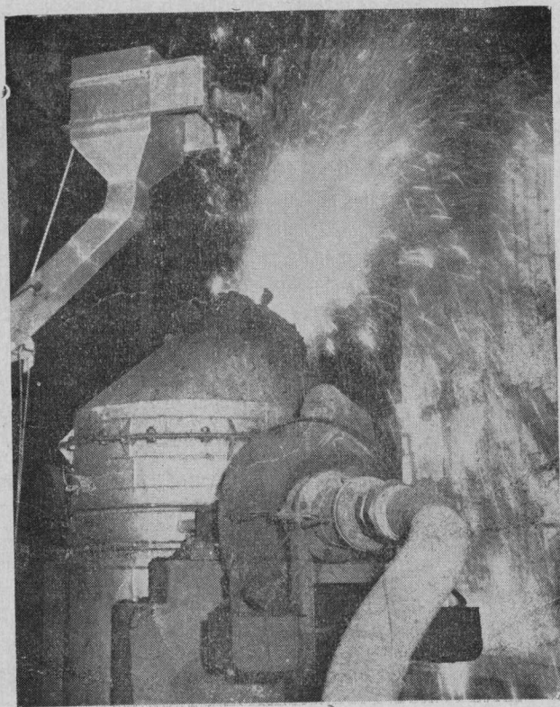
Basic Lined Side Blown Converter in operation,
